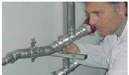
Figure 33 - Checking the press connection
