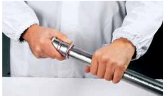
Figure 31 - Inserting pipe into the press fitting
