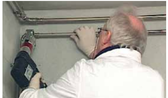
Figure 32 - Making the press connection
