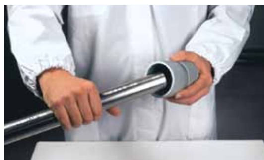
Figure 26 - Deburring the pipe
