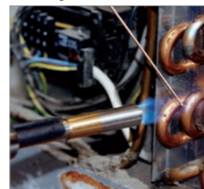
Brazing in aircon and refrigeration
