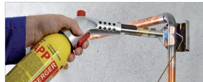
Brazing in gas installation
