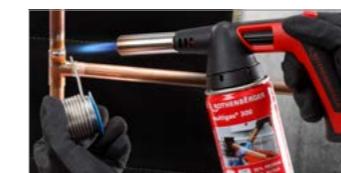
Soft soldering in drinking water and heating installation
