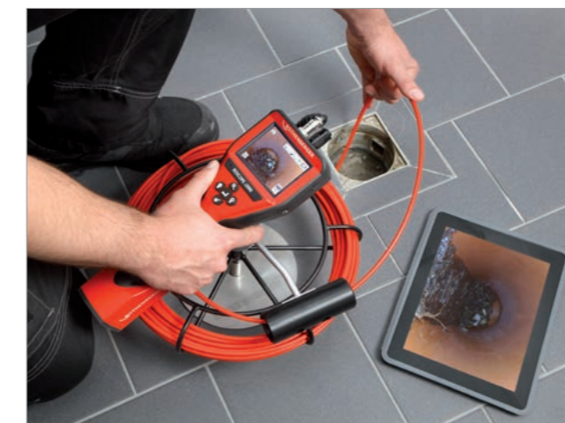
Inspection of basin drains
