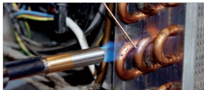
Brazing in aircon and refrigeration
