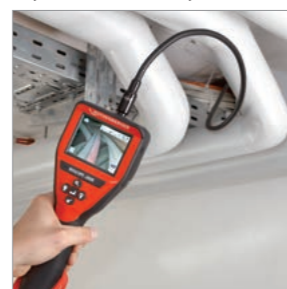
Inspection of hollow spaces
