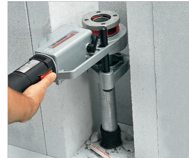
Work in confined spaces
