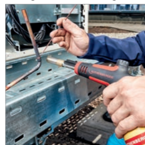
Brazing in aircon and refrigeration
