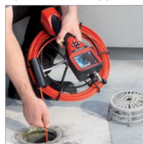
Inspection of rain downpipes
