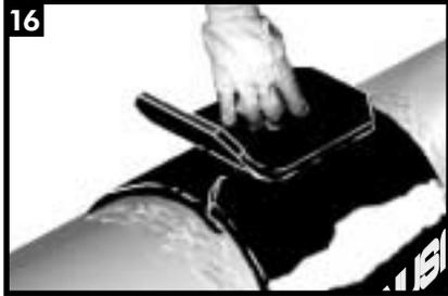
Remove the release liner from the hold down tape on the closure seal, centre it over the overlap and press it down.
