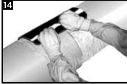
Centre the sleeve over the area to be sealed (casing pipe/PE pipe) and press the underlap into place. Remove the remaining release liner from the sleeve.
